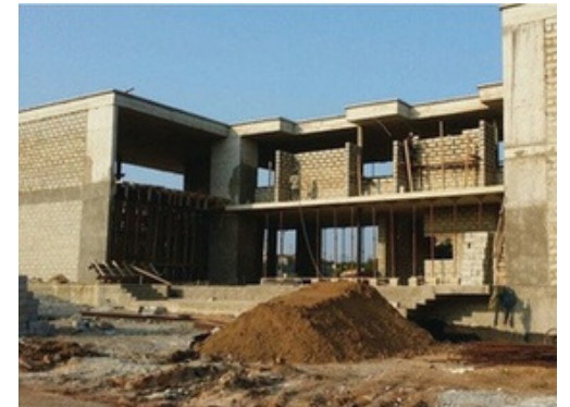
CASTING OF R F SLAB
