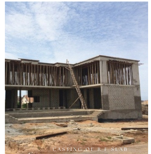
FORMWORK COMPLETE
