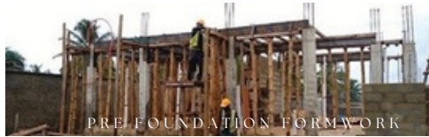
PRE FOUNDATION FORMWORK
